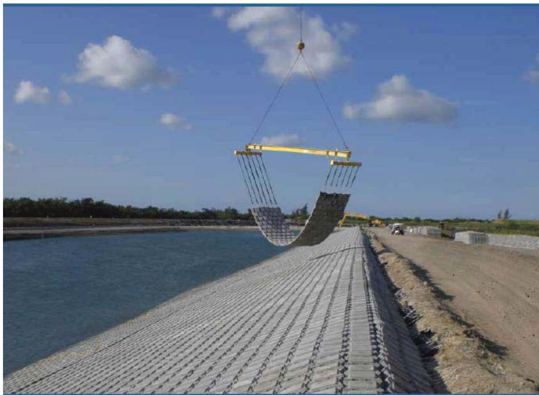
Figure 5.7-25. Typical Installation of Articulated Concrete Mat (Courtesy of CONTEC Engineering Solutions)
