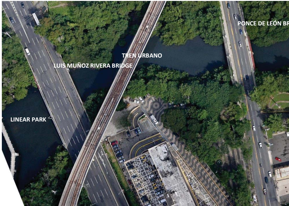
Figure 5.7-15. Channel Under Western Bridges
