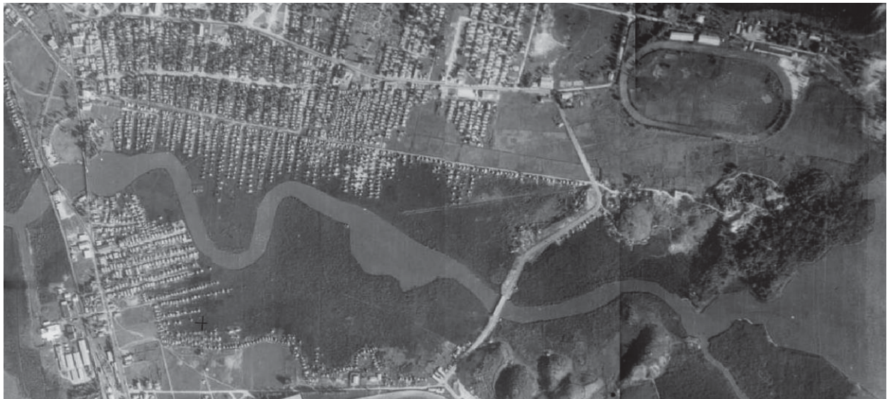
Figure 1.2-4. Historic aerial photo showing the conditions of the CMP in 1936
