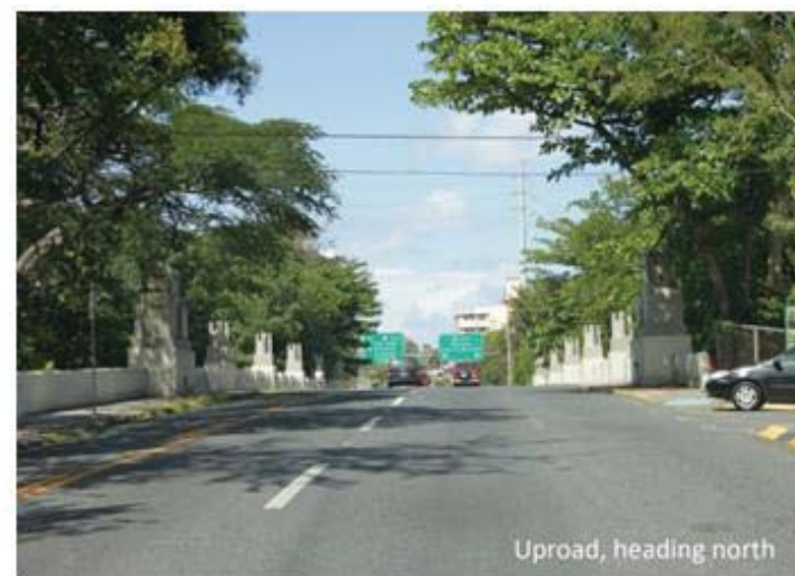
Ponce de León Avenue Bridge
