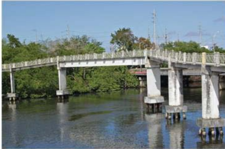
Linear Park Bridge
