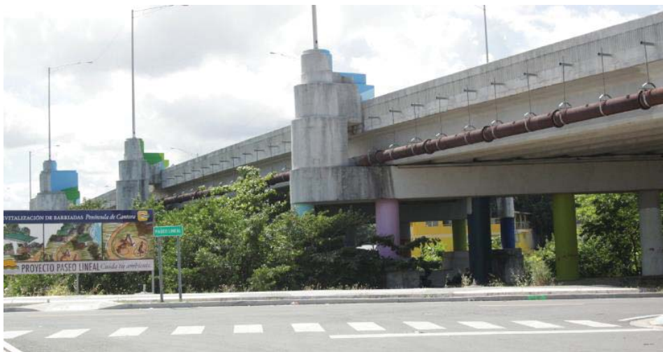
Figure 5.7-14. Channel Under Barbosa Avenue Bridge
